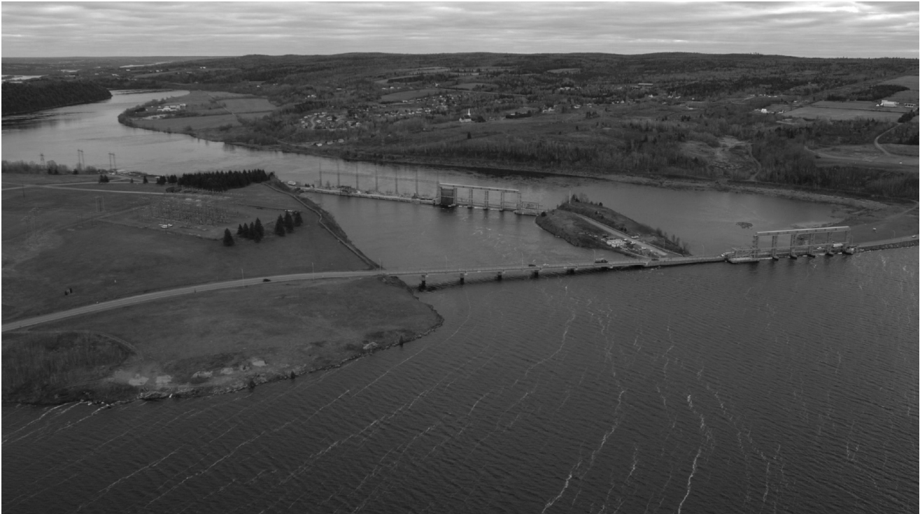
MACTAQUAC DAM — FROM THE WEST (2006)
