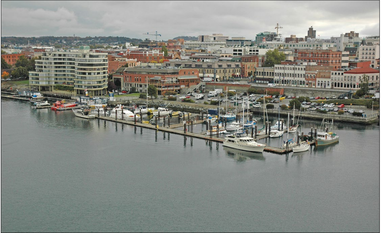
WHARF STREET MARINA (2005)
