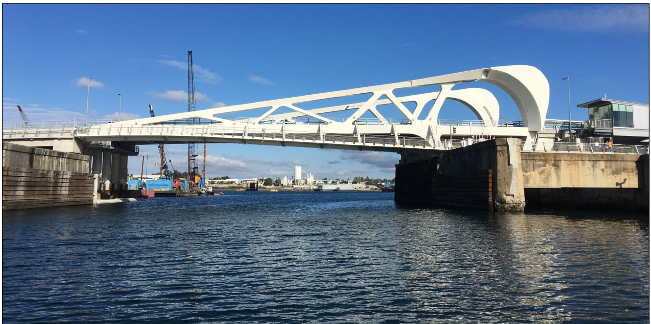
JOHNSON STREET BRIDGE — SPAN DOWN (2018)
