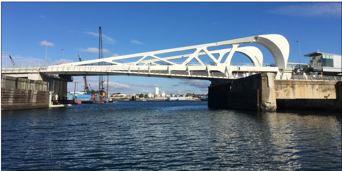
JOHNSON STREET BRIDGE — SPAN DOWN (2018)
