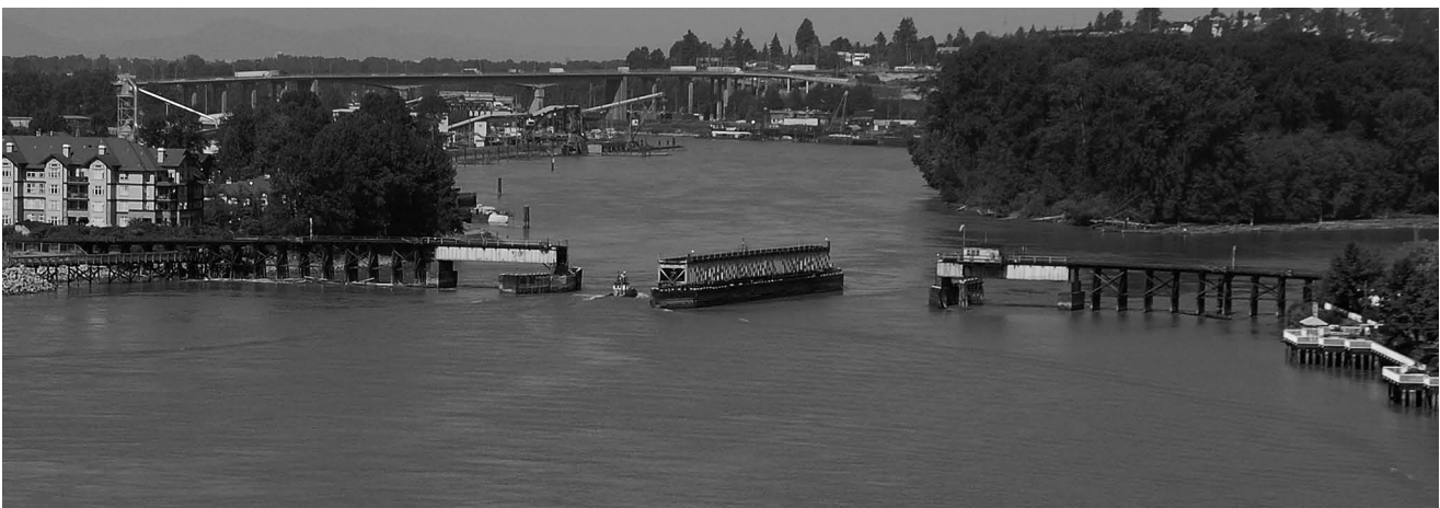
QUEENSBOROUGH RAILWAY BRIDGE (2007)
