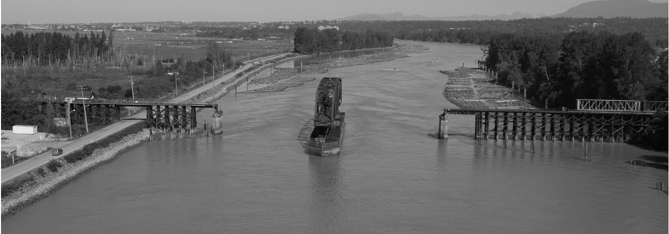
CANADIAN NATIONAL RAILWAY BRIDGE (2007)
