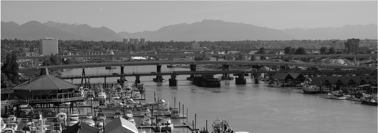
MIDDLE ARM SWING BRIDGE (2007)
