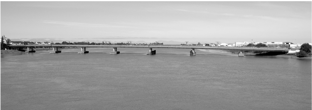
NO. 2 ROAD BRIDGE (2007)
