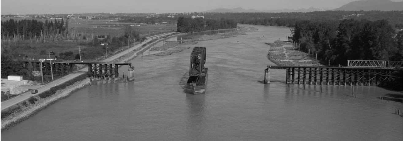
CANADIAN NATIONAL RAILWAY BRIDGE (2007)
