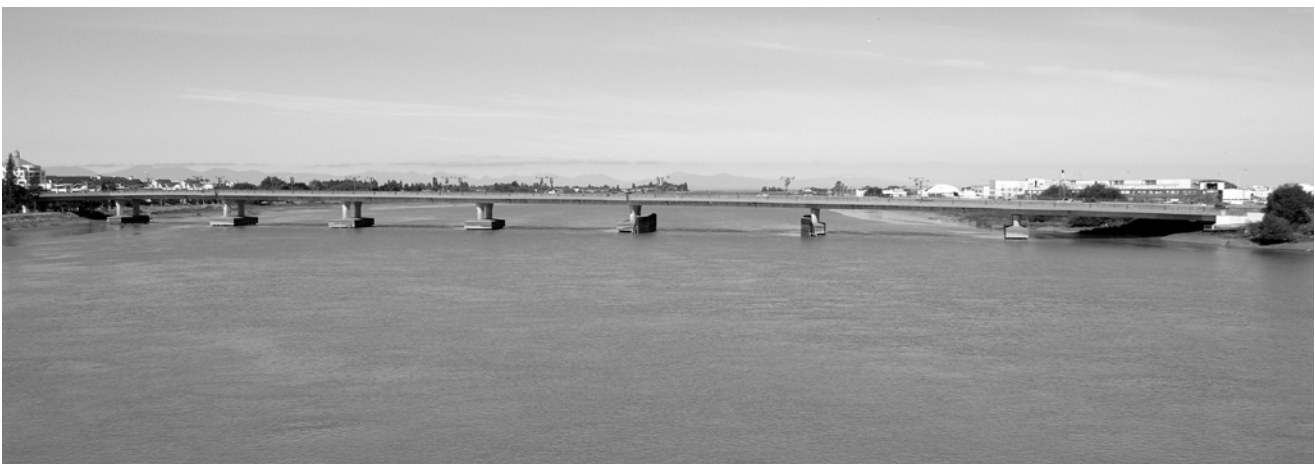
NO. 2 ROAD BRIDGE (2007)
