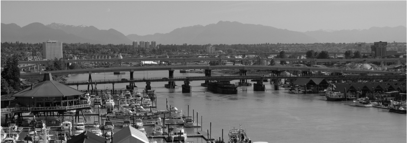
MIDDLE ARM SWING BRIDGE (2007)
