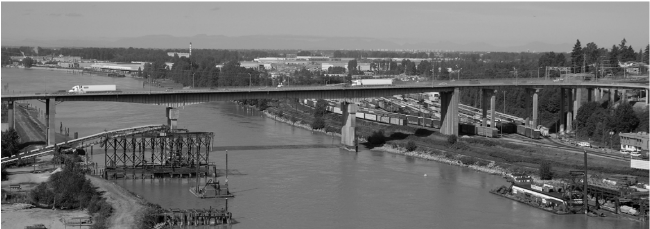
QUEENSBOROUGH HIGHWAY BRIDGE (2007)
