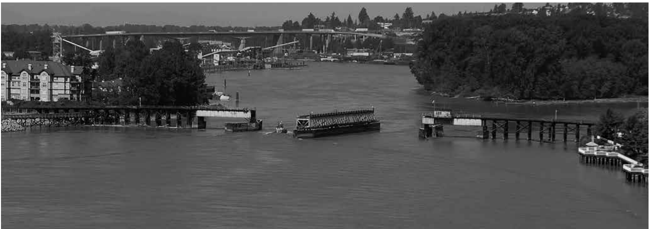
QUEENSBOROUGH RAILWAY BRIDGE (2007)
