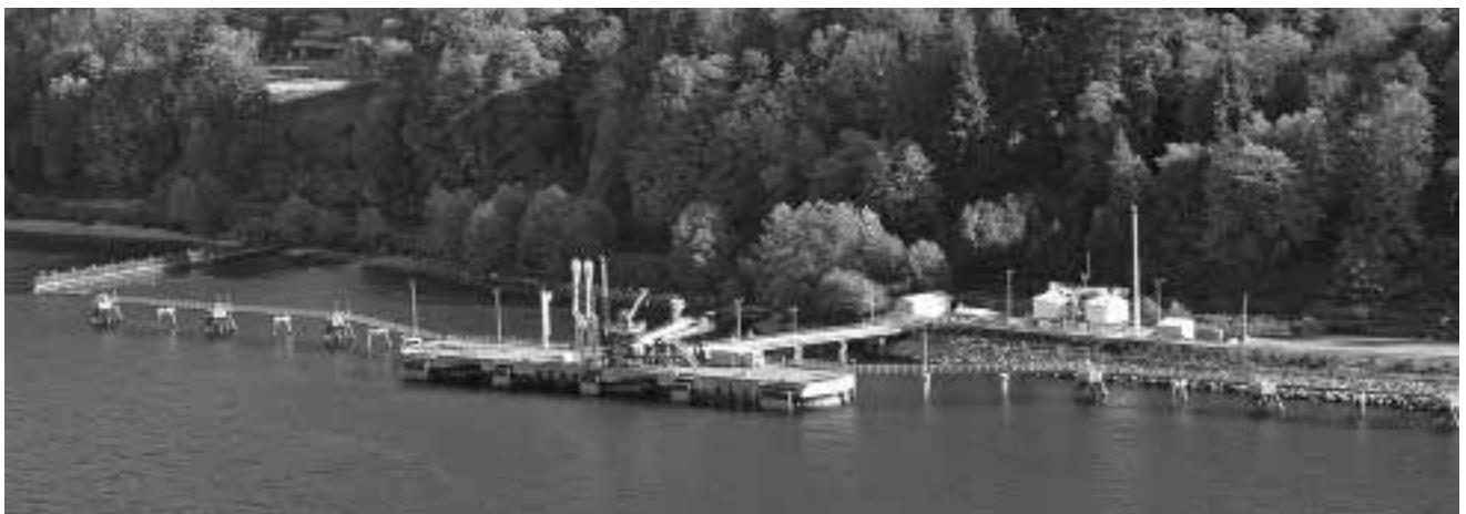
TERASEN PIPELINES WESTRIDGE MARINE TERMINAL (2005)
