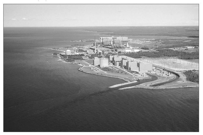
breakwaters are Y-shaped to reduce the surge effect in the basin.
