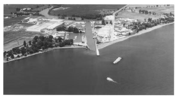
concrete breakwall extending 60 m (197 ft) offshore; the west pier is a shorter concrete and sheet steel wall with an elevation of 3 m (10 ft).
