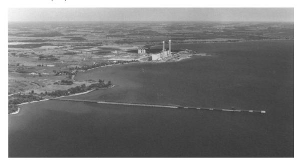
0.6 mile offshore; the berth is along the outer east face. It is a concrete structure with an elevation of 22 feet (6.7 m). There is a conveyor belt along the wharf and a hopper at the outer end. One hundred twenty-five (125) ships were scheduled for the 2015 season.
