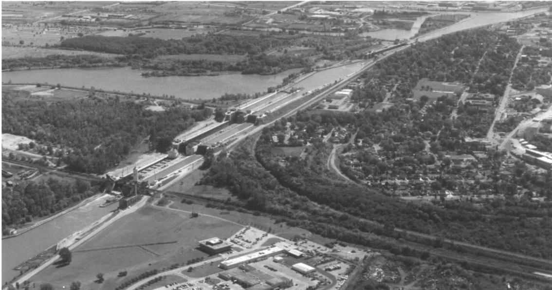
60 **Twin Flight Locks 4, 5 and 6** are entered 1 mile south of Lock 3. These three pairs of locks are stepped and raise vessels a total of 43 m (141 ft).
