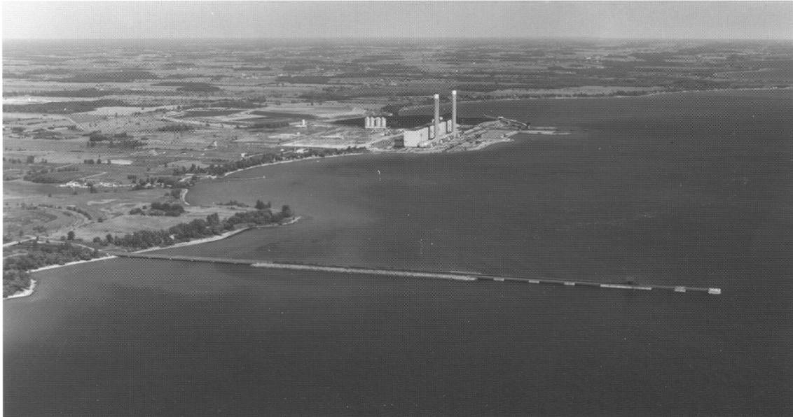
0.6 mile offshore; the berth is along the outer east face. It is a concrete structure with an elevation of 22 feet (6.7 m). There is a conveyor belt along the wharf and a hopper at the outer end. One hundred twenty-five (125) ships were scheduled for the 2015 season.
