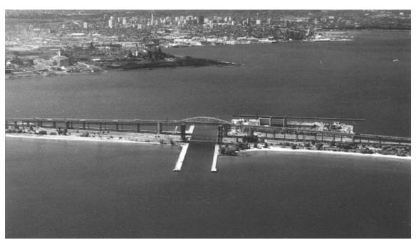
148 A **lift-bridge** and two high-level **bridges** cross Burlington Canal. The lift-bridge, near the mid-point of the canal, has a vertical clearance of 37 m (121 ft) when open and 3 m (10 ft) when closed. An overhead power line, with a clearance of 51 m (167 ft), crosses the canal 25 m (82 ft) NE of the lift-bridge. *Burlington Bay James N. Allan Skyway* Bridge, a twin high-level highway bridge with a vertical clearance of 38 m (125 ft), crosses the canal 135 m (443 ft) SW of the lift-bridge.
