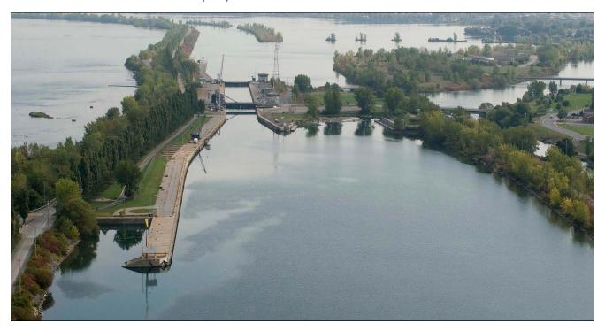
The main span of *Pont Victoria*, a combined road and railway bridge, crosses at the lower end of Saint-Lambert Lock; a diversionary road and railway **bridge** crosses at the upstream end. Each bridge has a vertical lift section with overhead clearances of 12 and 7 m, respectively, when lowered and 41 and 37 m in their raised position.
