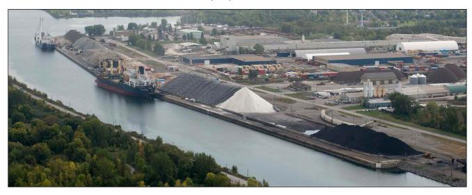
Côte Sainte-Catherine Lock has a lift of 10 to 11 m. The lower approach wall has a berthing length of 319 m; it is on the north side of the canal. Above the lock, the upper approach wall, also on the north side, has a berthing length of 318 m. Abreast of the approach walls the canal has been widened to 137 m. A bascule **bridge** spans the lock at its upstream end.
