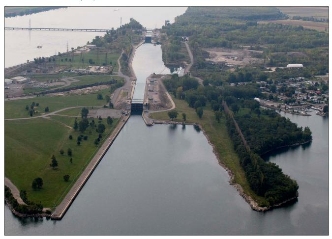
approach wall, on the east side of the channel, has a berthing length of 379 m. A tunnel under the lock carries traffic between Beauharnois and Melocheville. The upper approach wall is on the east side of the channel above the lock. The lock and approach walls are illuminated at night.
