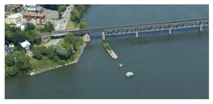
57 **Pont Beloeil**, a railway fixed bridge  $(45^{\circ}33'N, 73^{\circ}13'W)$  with a vertical clearance of 10 m, crosses the river at McMasterville.
