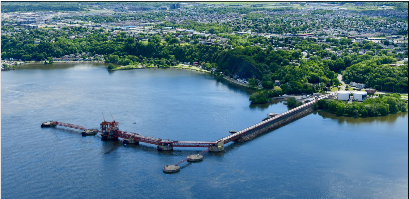
VALERO ENERGY REFINERY PETROLEUM TERMINAL (2019)
