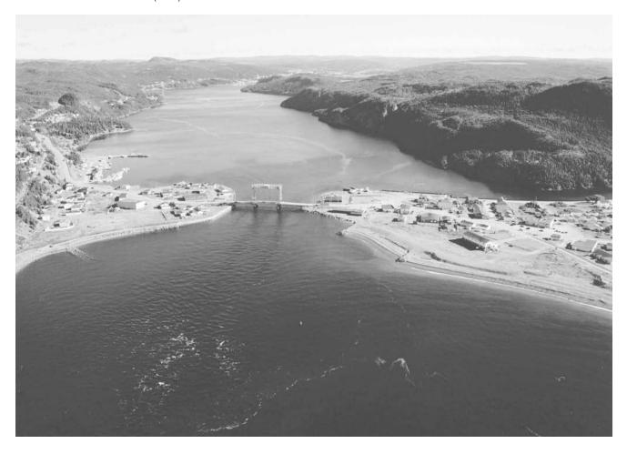
Bridge. — The channel under the vertical lift-bridge spanning Placentia Gut is 26 m (85 ft) wide. When the bridge is open, there is a vertical clearance of 21.3 m (70 ft), and when closed, it is 3.7 m (12 ft). Vessels requiring the bridge to be opened should contact the bridge-master on VHF radiotelephone channel 10 (156.5 MHz) or by telephone at (709) 227-2154. If radio contact is not made, three long blasts should be sounded on a whistle or siren.
