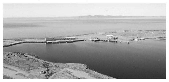
Close north of the ferry wharf is the Marine Atlantic coastal wharf, (Berth 6), which has a berthing length of 31 m (102 ft) with depths of 1.2 to 4.3 m (4 to 14 ft) alongside its outer 20 m (66 ft) length. The deck of this wharf has an elevation of 1.5 m (5 ft).
