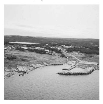
A stone breakwater 37 m (121 ft) long is located in the SE corner of the harbour. A slipway is located close south of this breakwater.
