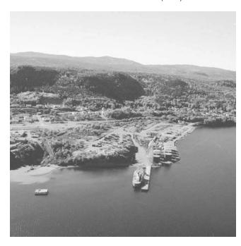
155 The Clarenville Drydock wharf, situated close north, has dimensions similar to the previous wharf and a depth of 4.8 m (16 ft) at its outer end. A marine railway with a capacity of 600 tonnes is located on the north side of this wharf. Fresh water and electric power are available at this facility (See Appendix).
