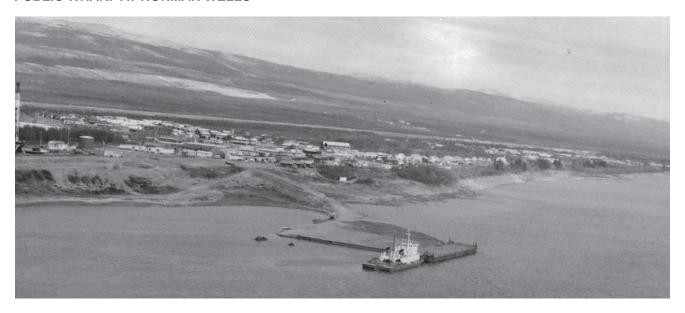
An ESSO fueling wharf, 51 m long at the outer face, is 0.2 mile downstream from the Public wharf. The depth alongside is 2.7 m. Northern Transportation Company Limited (NTCL) loads various types of fuels on its barges here for transport north. NTCL has an office near the Public wharf. Another wharf, serving the Imperial Oil Company refinery, is 0.7 mile west of the fueling wharf.
