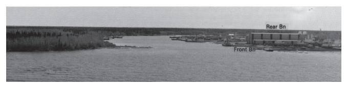
East Channel (60°50′N, 115°45′W) of Hay River is approached through a dredged channel, 122 m wide and almost 0.7 mile long. The dredged channel is reported (1972) to be maintained to a depth of 2.4 m, sand and mud bottom. Inside the approach channel East Channel provides a natural harbour with numerous marine facilities along its west bank.
