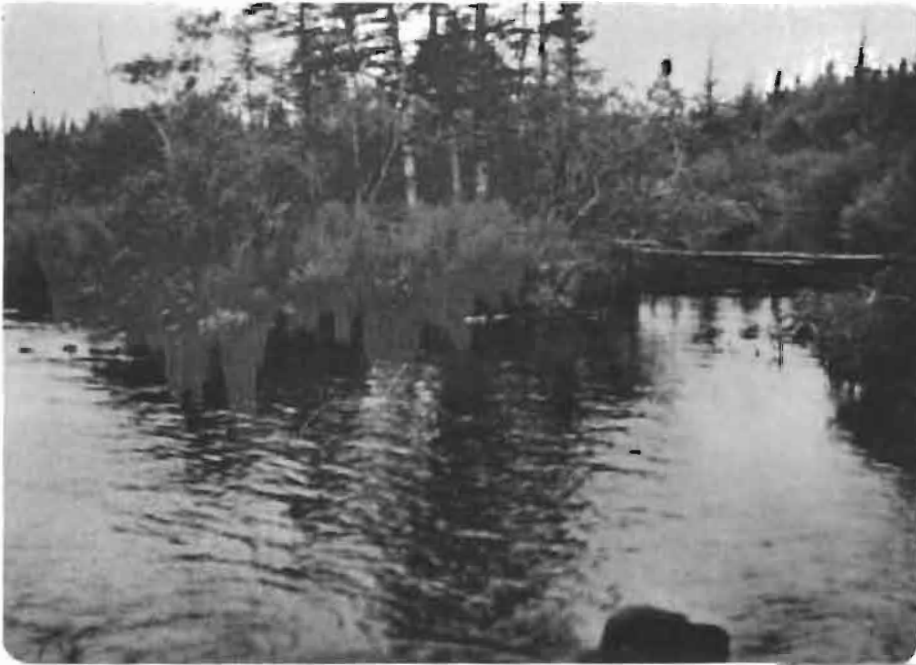
Photo No. 7 - River run-around before construction.
