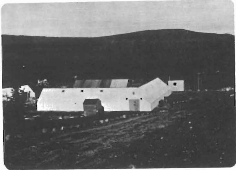
Photo No. 13. Overall view of the hatchery, summer, 1977.
