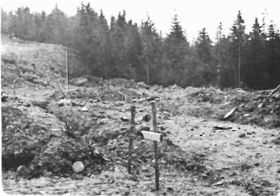
Photo No. 2 - Early road construction to site.
