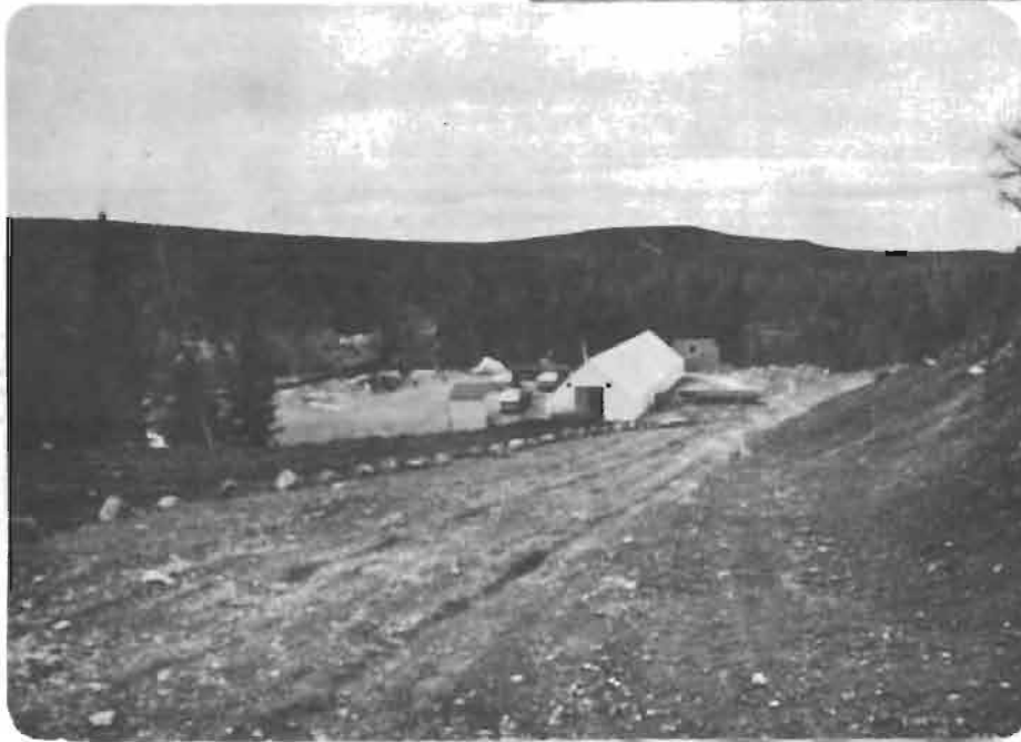
Photo No. 5 - Hatchery building, Spring, 1977.
