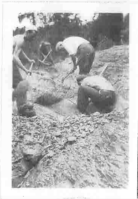
Figure 2. Construction work on minor fishway.
