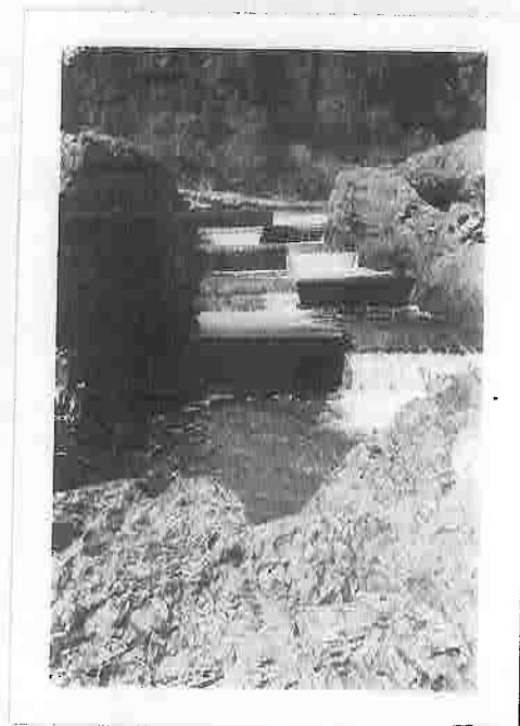
Figure 7. Fish ladder at low water. July 20, 1937.
