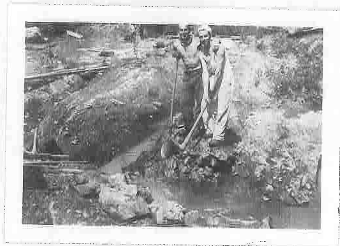
Figure 3. Construction work on major fishway.
