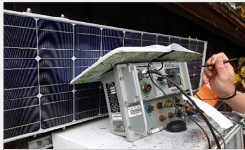
Real time water temperature logger installation on Stuart River.
