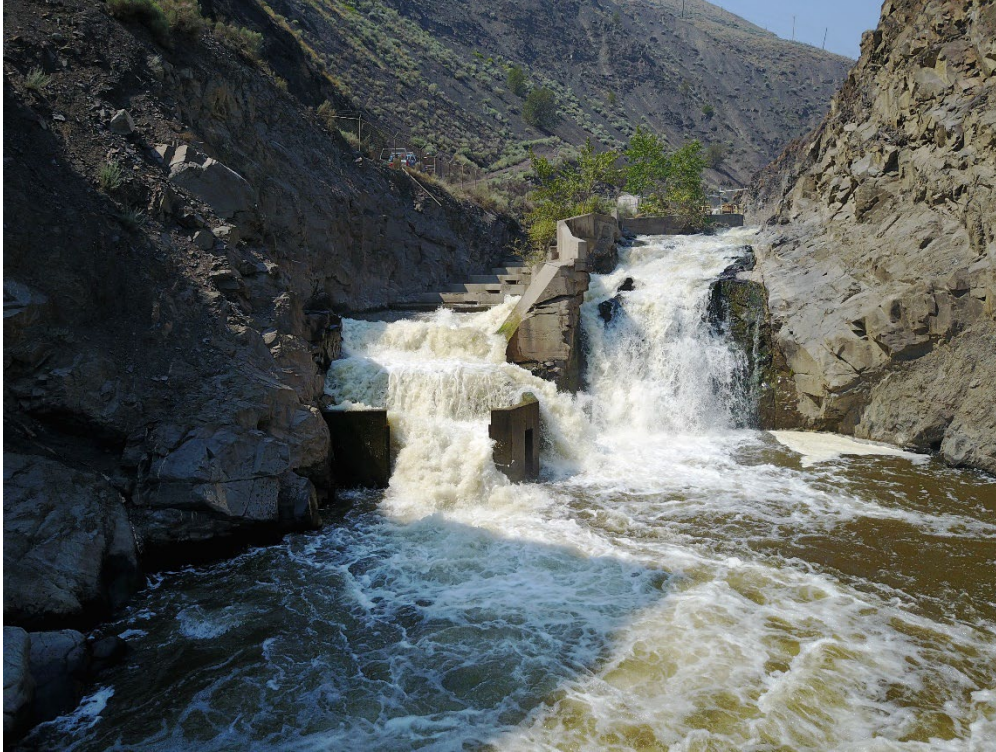
Figure 22. Bonaparte Fishway that facilitates upstream Chinook migration.
