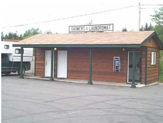
Sointula Washroom Facilities
