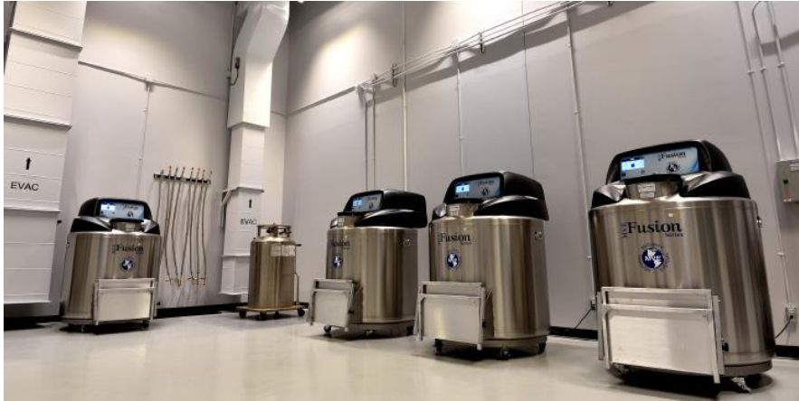
Figure 1. Some of the installations at the National Biodiversity Cryobank of Canada located within the Natural Heritage Building of the Canadian Museum of Nature, on 1740, Pink Road, Gatineau, Québec. This is where tissue samples, including mantle biopsies, of freshwater mussels can be stored in liquid nitrogen ( -185^{\circ}\text{C} ) for curation and archiving for posterity. Photo credit Canadian Museum of Nature.
