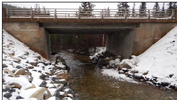
c) Pont permanent
