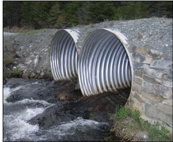
Figure 3.21 Multiple culvert installation.
