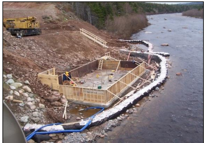
Figure 3.37 Cofferdams can be used to isolate stream margin work areas from stream flow.
