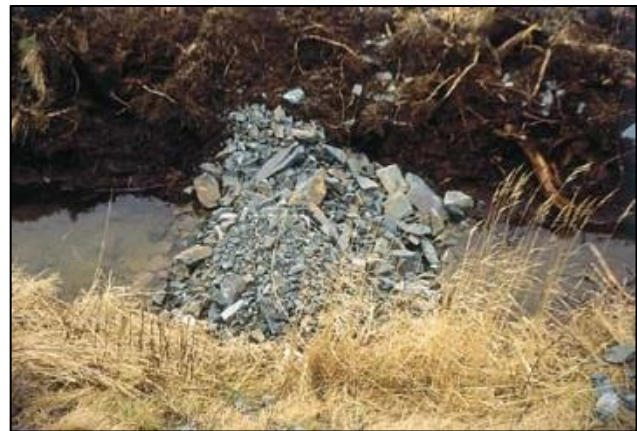
Figure 3.5 Check dams can be constructed from a variety of readily available materials, including rocks.
