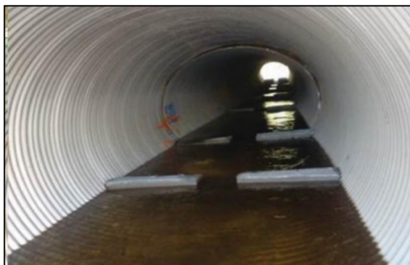
Figure 3.25 Culvert baffles.
