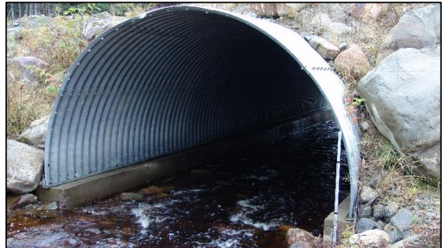
d) Bottomless arch culvert installation.
