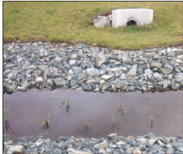
Figure 3.15 Rock riprap prevents erosion.
