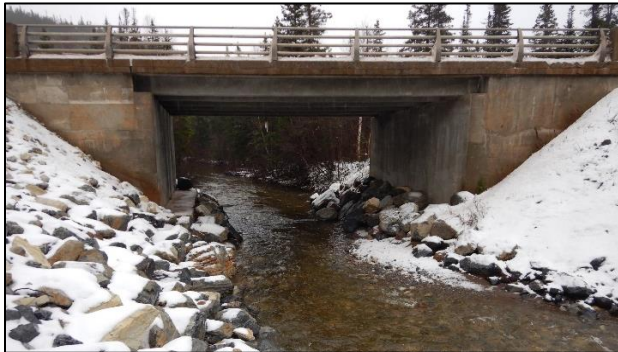
c) Permanent bridge.
