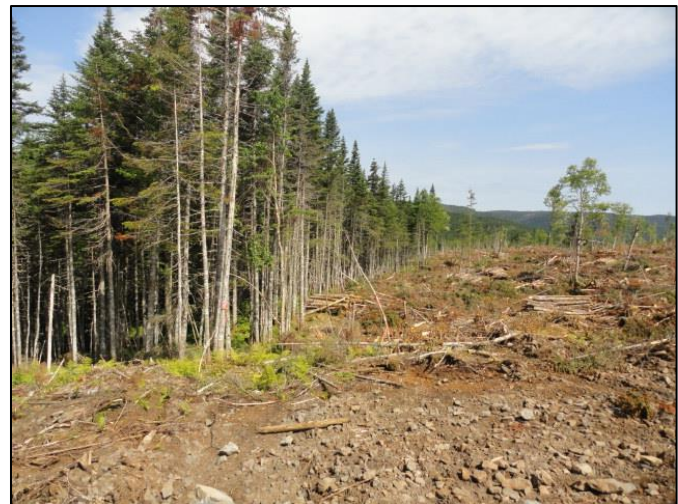
Figure 3.35 Right-of-way clearing and grubbing is commonly associated with many construction developments, including roads, pipelines and transmission lines.
