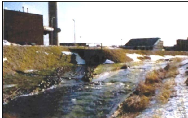
Figure 3.44 Storm drainage outlets should be connected to the receiving watercourse by a channel with orientation parallel to the flow of the receiving watercourse.
