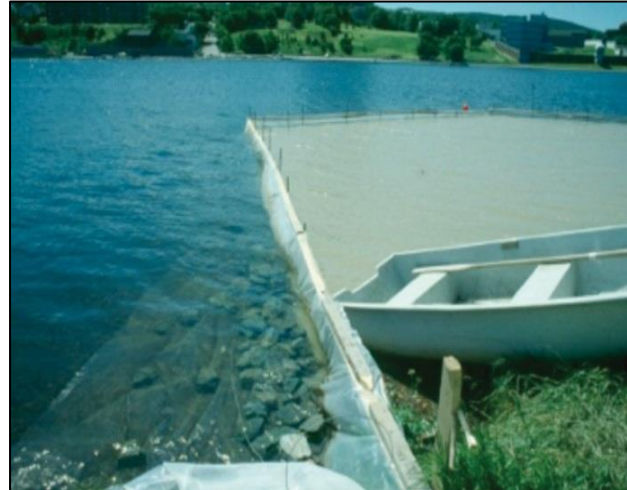
Figure. 3.46 Suspended curtain to contain suspended sediment in immediate work area.
