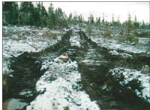
Figure 3.48 Mudlogs divert water off of the trail and onto the forest floor
