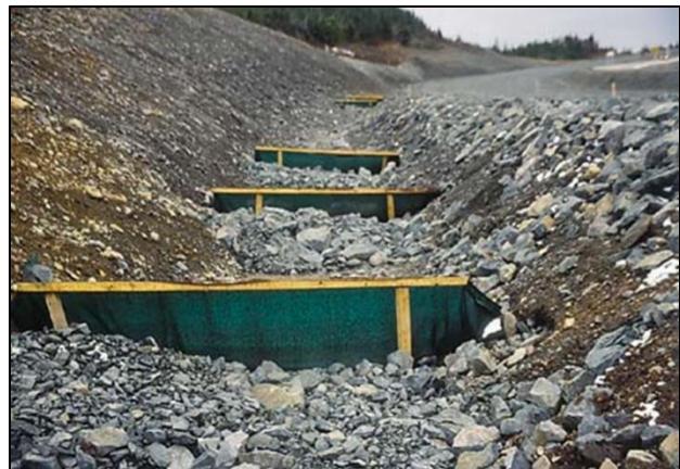
Figure 3.3 Filter fabric dams installed in series.
