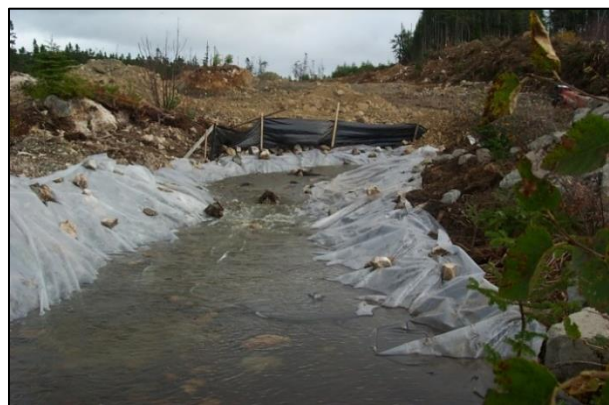
Figure 3.9 Settling ponds should be lined with an impermeable material, such as plastic, to prevent the generation of silt from the excavated settling pond.
