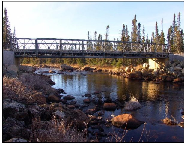
Figure 3.17 A well-designed bridge allows for a natural stream bottom at a crossing site.
