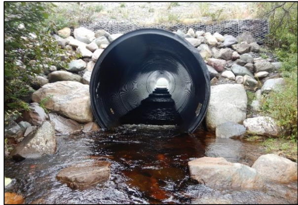
Figure 3.20 Countersunk culvert.
