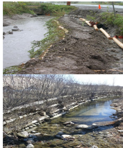
Figure 2. Riparian shoreline works during construction (top), and after completion (bottom). Photo credit: DFO.
