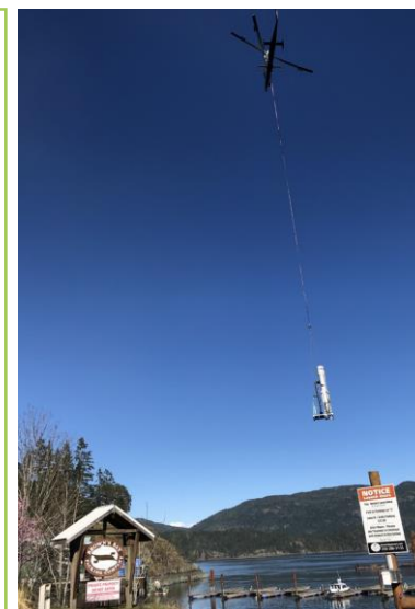
Fluidized Bed Reactor being airlifted into position at a wastewater treatment plant.
