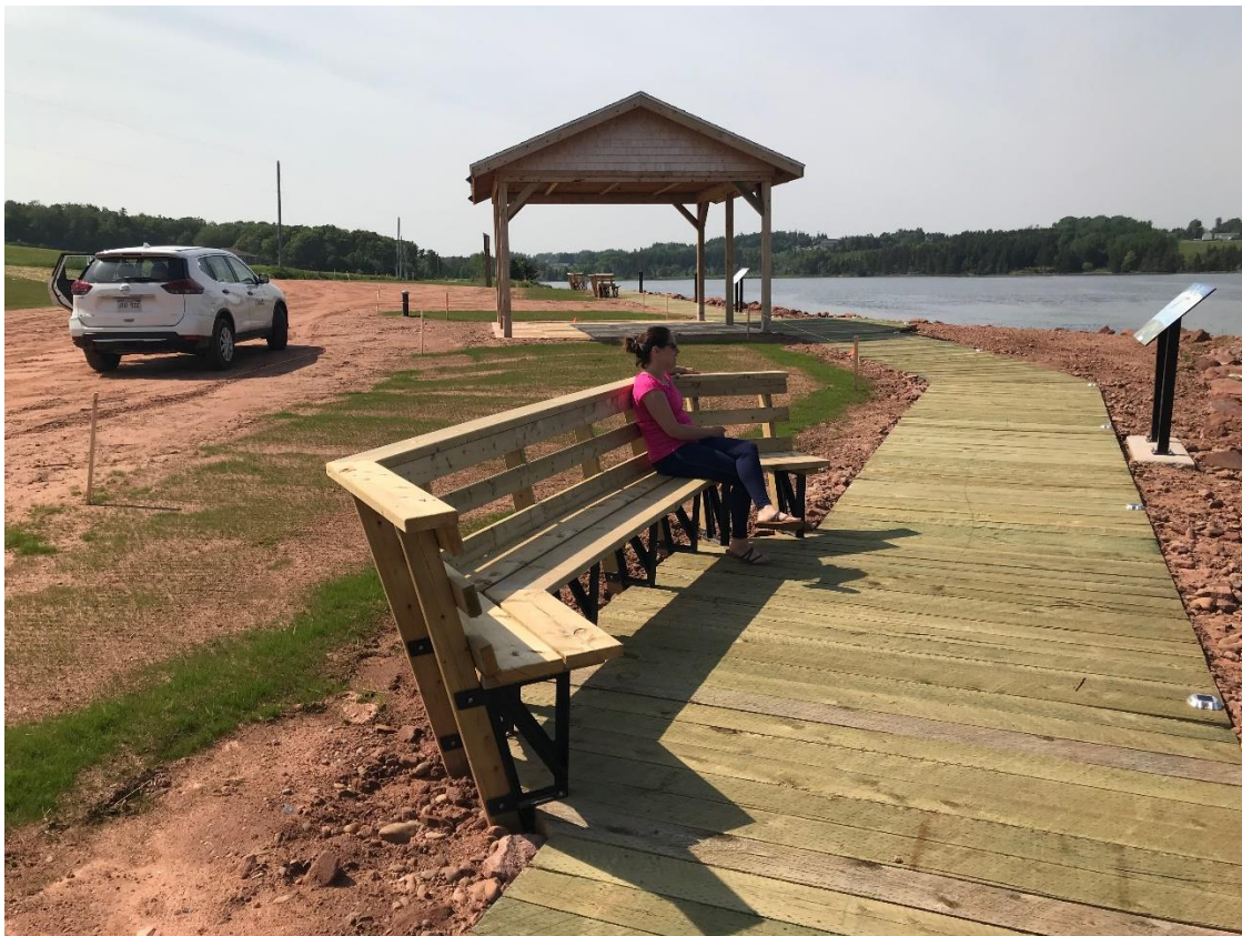
Figure 5. New Gazebo and boardwalk with interpretive panels at the Basin Head Interpretive Park.
