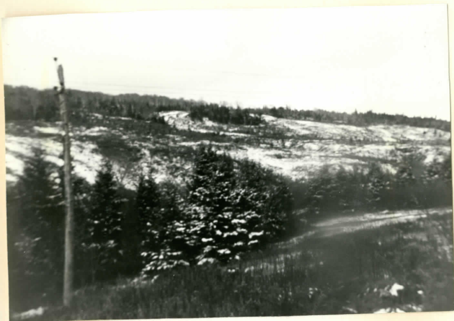
Photo 3. River Valley at Ogden Showing Results of Heavy Wood Cutting.
