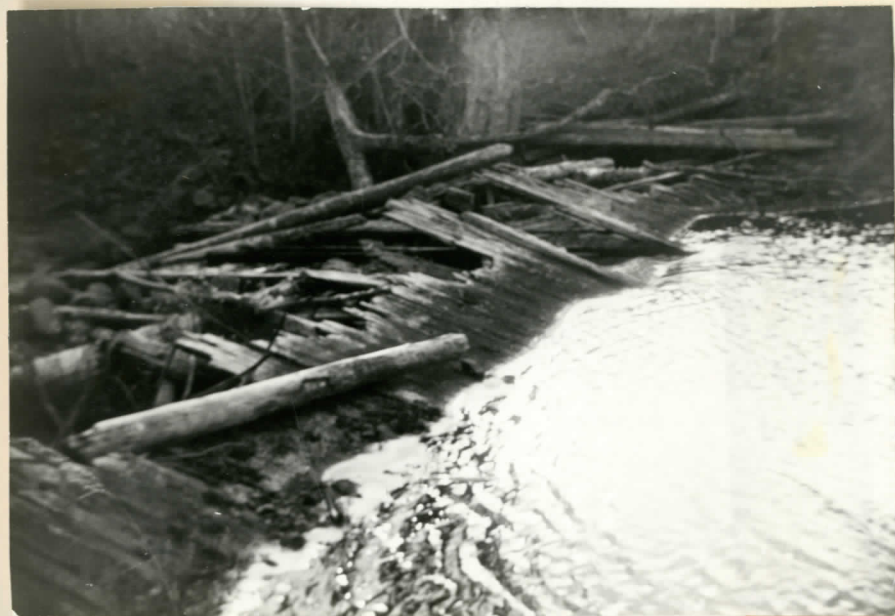
Photo 10. Remains of Dam (breached) at Foot of Sullivan's Lake. About 17 Miles Upstream.
