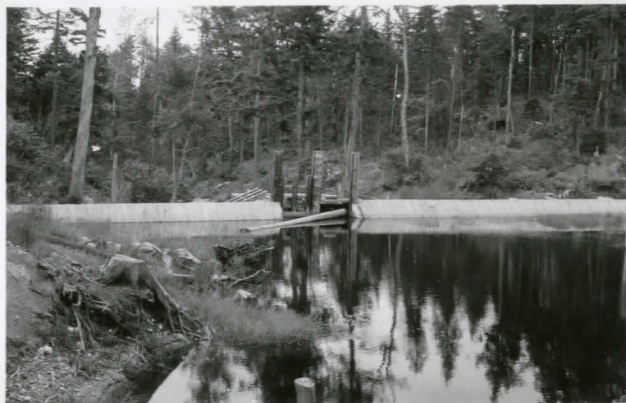
B-7. Timber Lake Dam
