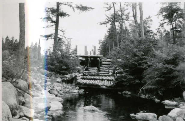
B-7. Timber Lake Dam
