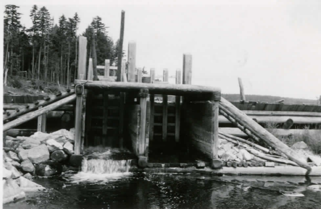
B-6. Coolan Lake Dam
