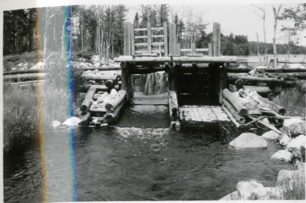
B-5. Bad Lake Dam
