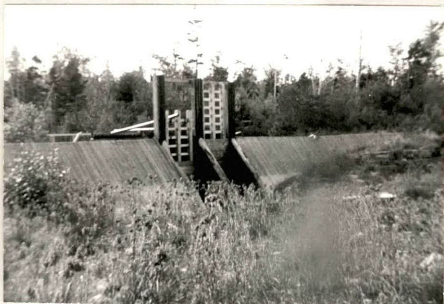
Photo 16. Former driving dam at Long Lake in the headwaters of the main river.
