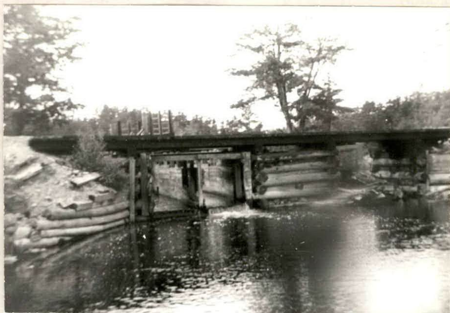
Photo 17. Former driving dam at Hendry Lake in the headwaters region on the West Medway River.
