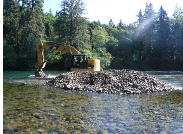
Figure 2. Gravel placement for Chinook salmon spawning in the Campbell River, 2018. Photo credit: Shannon Anderson (DFO)
