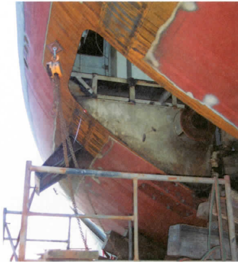
Two large holes are cut into the side of the ship for installation of the fins
