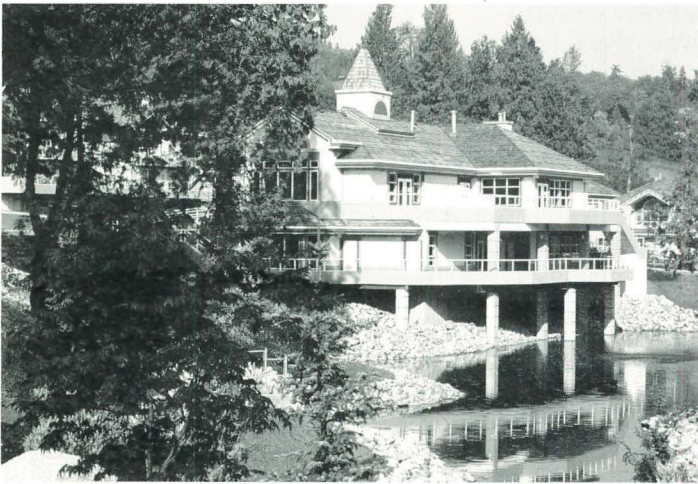
Incorporated as a feature of the new development, this lake is the key to sediment and erosion control, acting as permanent silt retention, storm detention and flood control facility.
