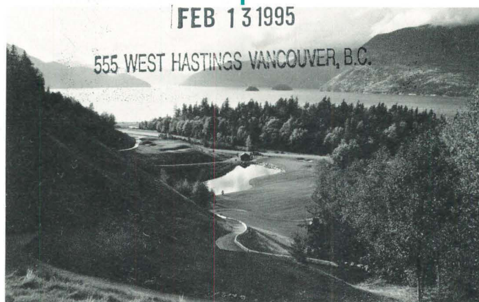
The steep hillsides of Furry Creek development show the necessity for erosion and sediment control. Looking down from a golf tee on high shows how the control pond fits in with the overall design. This pond also serves as an organically balanced irrigation source for the course.
