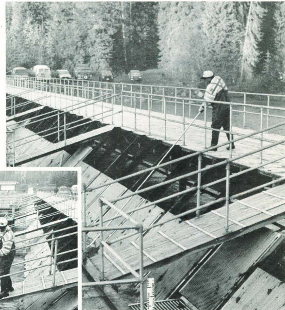
Fish carcasses and leaves are removed as they wash up on the fence, a 100-metre structure spanning the width of the Babine River. Inset: Jim Hansen and Ian Bergsma record the number of salmon which pass through the fence's seven traps.
