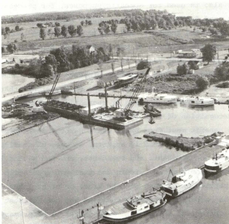
Wheatley Harbour Under Construction
