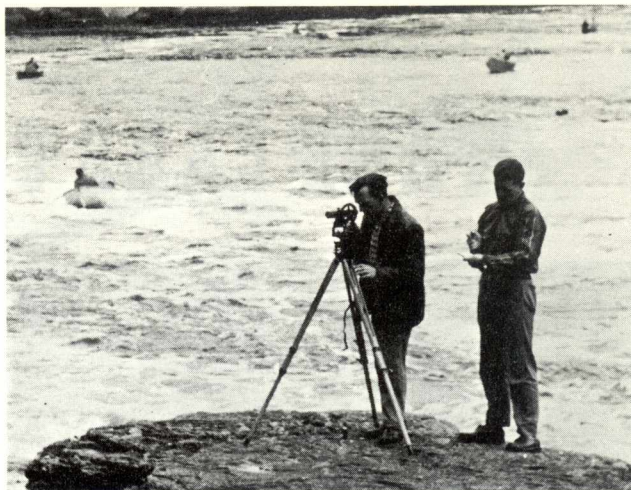
Engineering Survey Crew, Big Falls, Humber River, Nfld.
