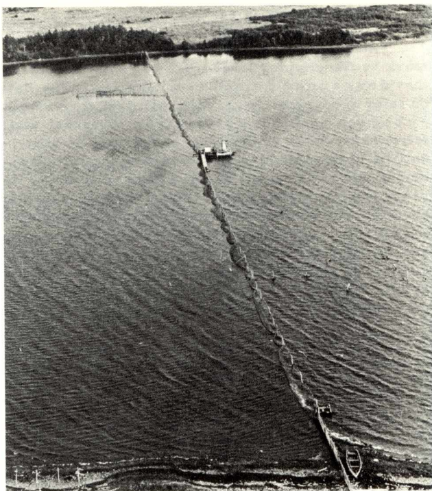
Aerial view of salmon counting fence, Little Codroy River, Newfoundland; downstream is to right, and tide is running in, with on-shore breeze causing nets to billow upstream. Trap for seaward migrating smolts and stage for fish examination and marking are in middle distance; traps for upstream moving adults are in background to left of barrier nets and in foreground to right of barrier nets.
