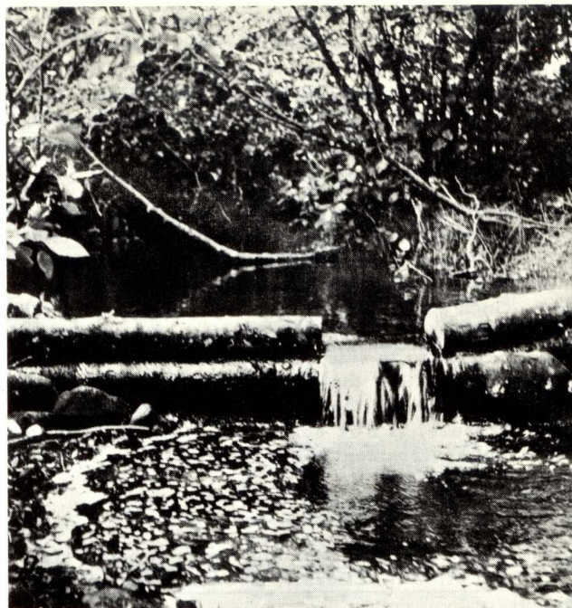
Stream improvement by construction of low dams to provide more living space (pool formation) for brook trout. Ellerslie Brook, Prince Edward Island.
