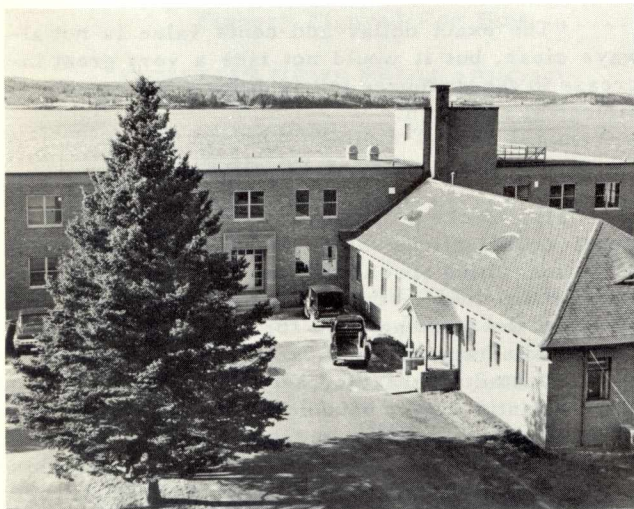
The new wing at the St. Andrews Station, with one of the older buildings in right foreground.
