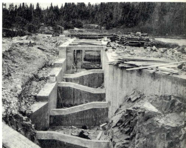
Fishway under construction
