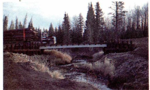
Stream crossing on a logging road in Alberta. This well-designed crossing left the stream in a natural condition.
