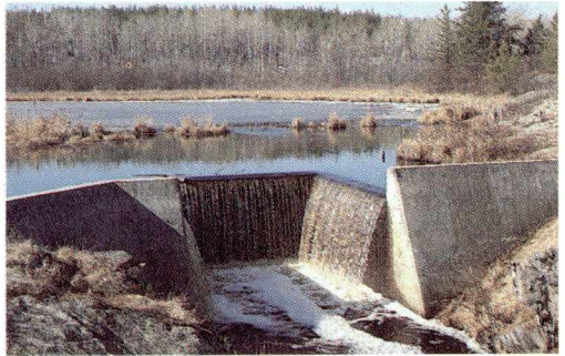
Weir near Caddy Lake in Manitoba. It acts as a wall, blocking fish movement to upstream spawning areas.
