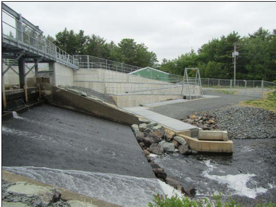
Figure 6. Fish passage facility at Hebb Dam on the Petite Rivière.
