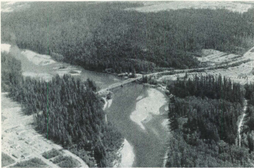
Highway bridge at Kitimat Center
