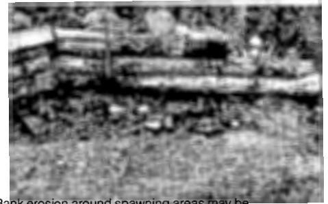
Bank erosion around spawning areas may be controlled using stop-logs. This work was done by a Nanaimo citizens group.
