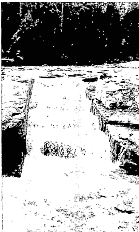
The Nib Falls vertical-slot fishway was partly constructed using explosives to create smooth rock faces.
