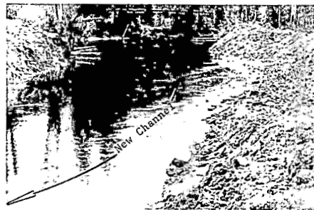
Bypass channels may be constructed around large obstructions, like this one around a log jam on the Nahatlatch River.
