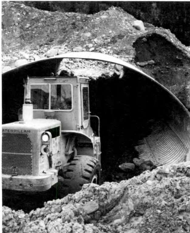
Construction of the huge culverts on the Rose River crossing was a major habitat concern in Yukon.
