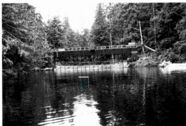
Counting fence on the Docee River for enumerating salmon escapements.
