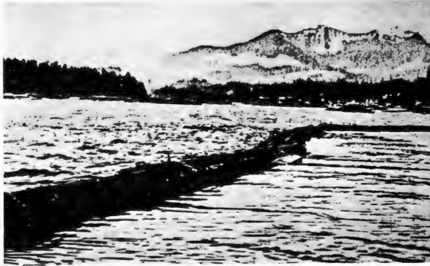
A. Floating log bundle breakwater
