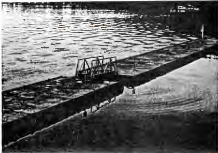
A. Floating Caisson breakwater of 4.6 m width and 1.1 m draft at Friday Harbour
