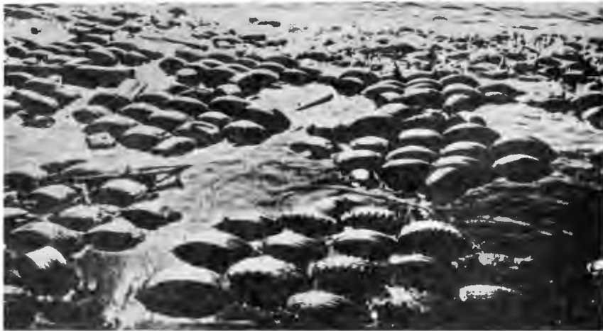
B. Goodyear module design breakwater at North Vancouver, B.C.
