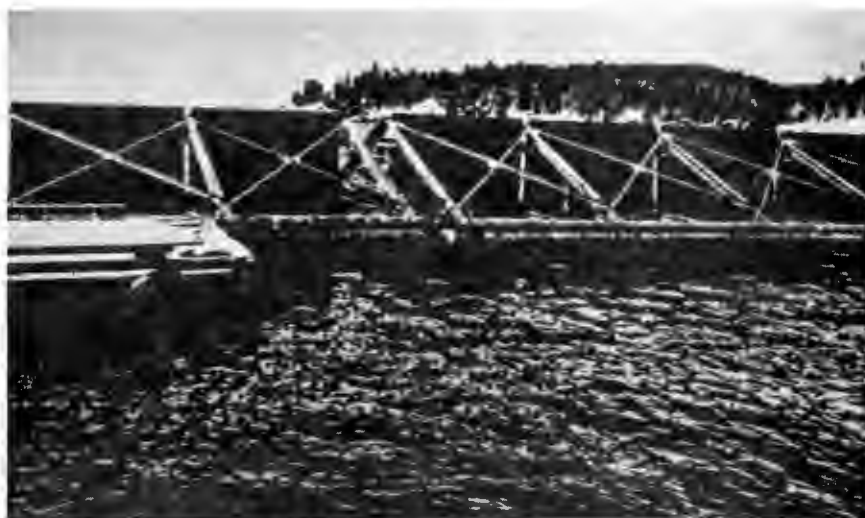
B. Lund A-Frame breakwater construction
