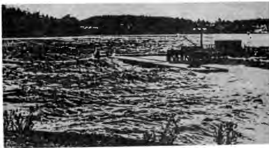
B. Friday Harbour breakwater in 2.8 sec. waves
