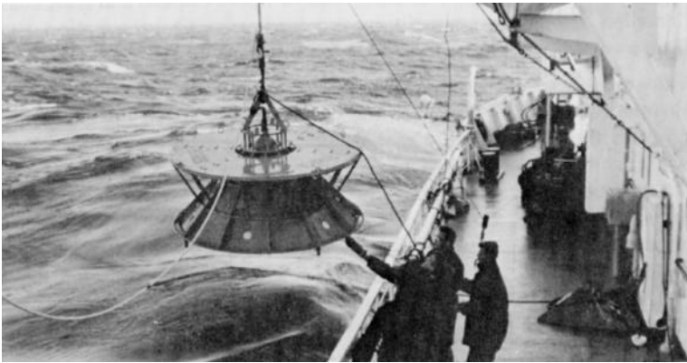
Hudson's deck crew recovering a directional hydrophone in the Atlantic for scientists from the Defence Research Establishment Atlantic: The hydrophone was used with explosive sources to study scattering from layers of fish at depths up to 1000 metres.
