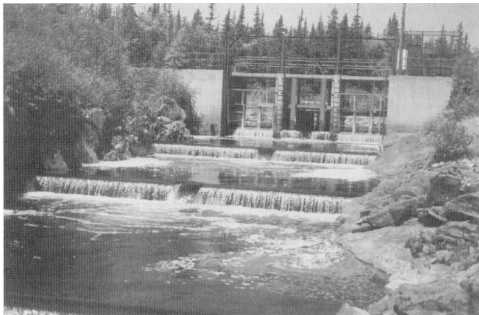
Fish trapping facilities at upper end of the Liscomb River fishway
