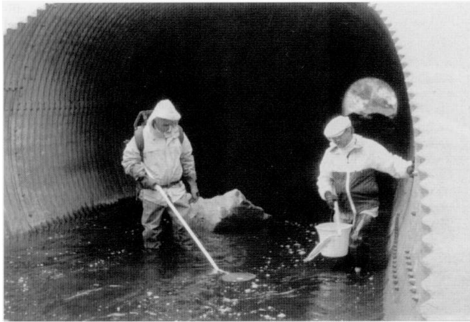
Jim Leadbetter (left), Habitat Management Branch, and Vern Conrad, Biological Sciences Branch, electroseining in a natural bottom culvert.
