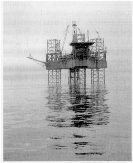
Cohasset/Panuke offshore drilling platform
