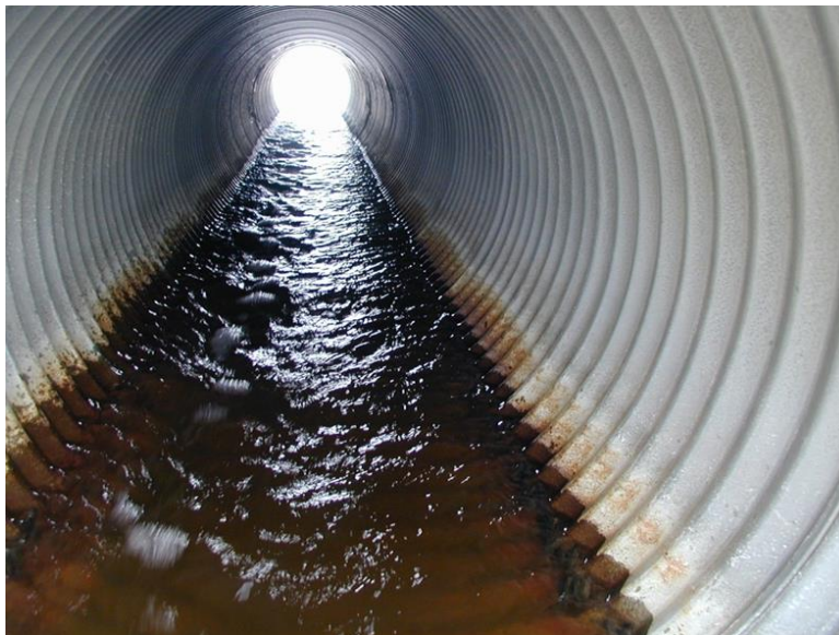
Figure 4. Field studies with culverts and fish passage.
