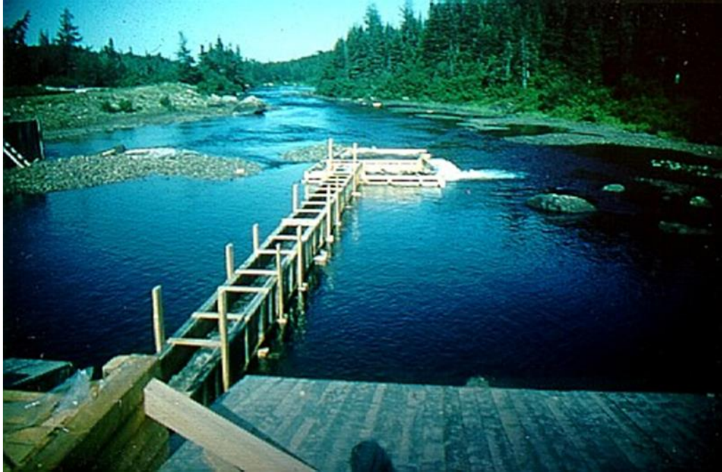
Figure 2. Temporary Ecohydraulics Flume (channel or raceway) in NL
