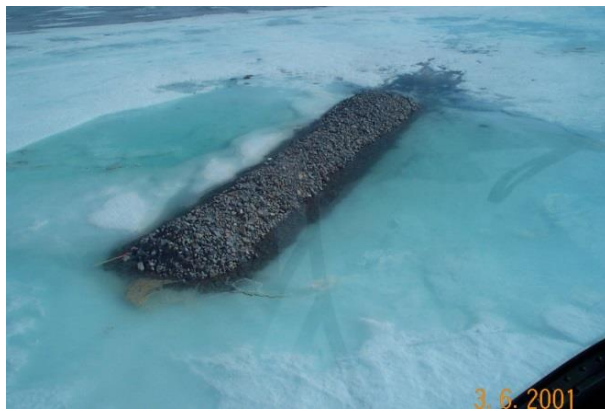
Figure 6. Snap Lake showing a) the transport of rock out onto the ice, b) the final reef profile on the ice and c) the initiation of the reef subsidence at ice out.
