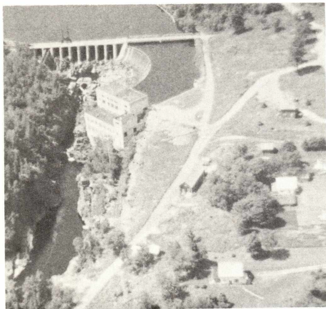
Aerial view of Nepisiguit River's Grand Falls hydroelectric development, showing horse-shoe spillways and deep gorge below.
