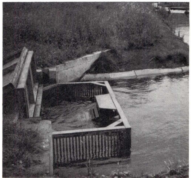
Recovery trap for salmon returning to Mactaquac Hatchery release channel.
