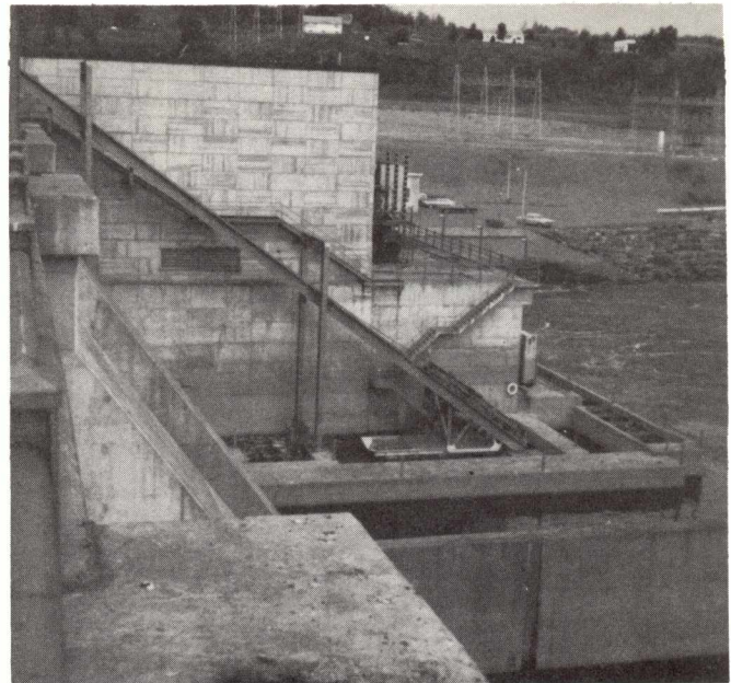
Overall view of fish lift facilities at Beechwood Dam.
