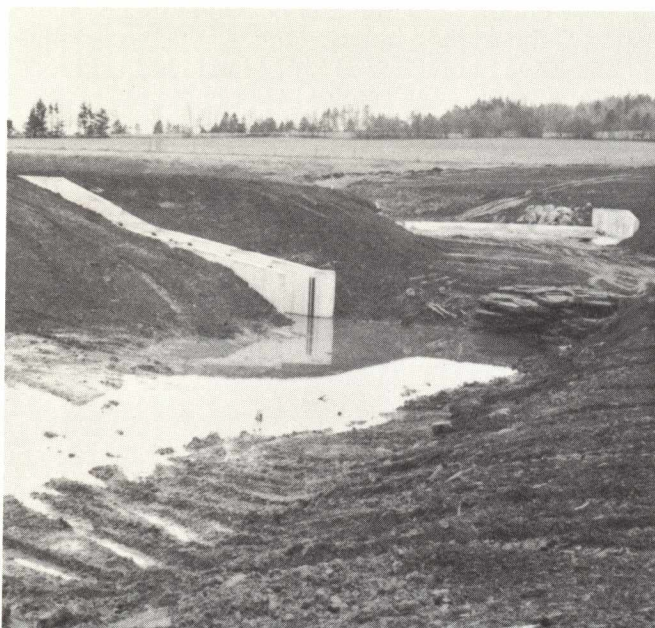
Construction of Bell's Pond fishway, Prince Edward Island.
