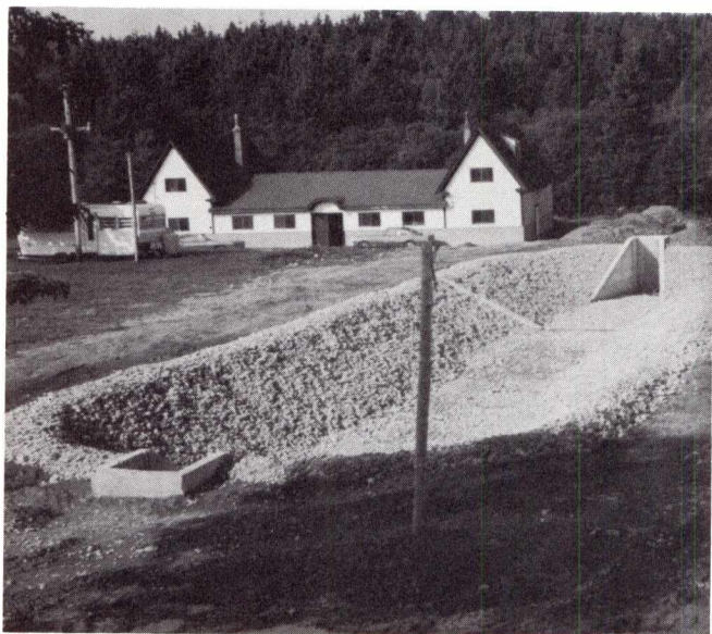
New salmon broodstock pond under construction at Antigonish Hatchery.
