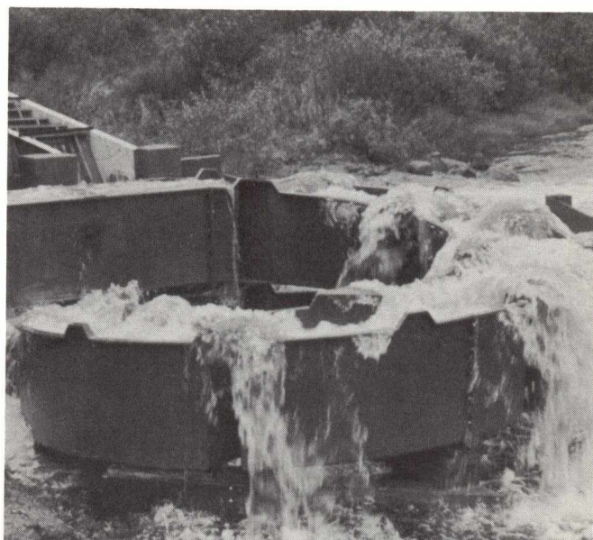
Spiral fishway under high water conditions at Oxford Junction, River Philip, Nova Scotia.
