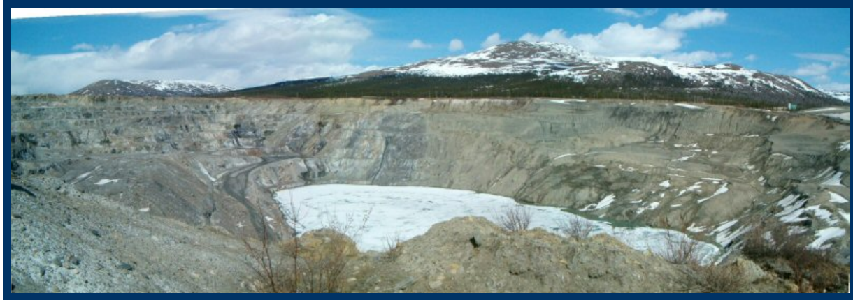
The Vangorda Mine pit on the Vangorda plateau; part of the larger Faro Mine complex
