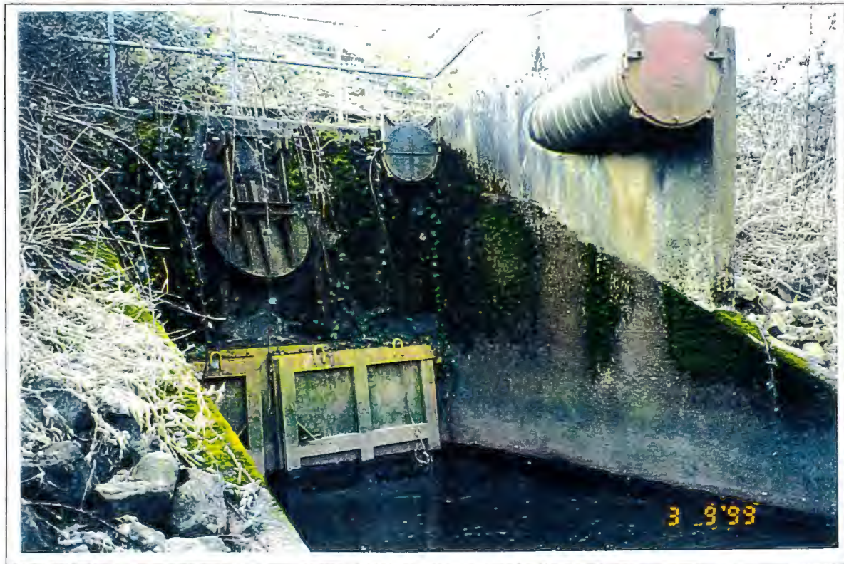
Photo 18: Nathan Slough station: flood box and pump outfalls.
