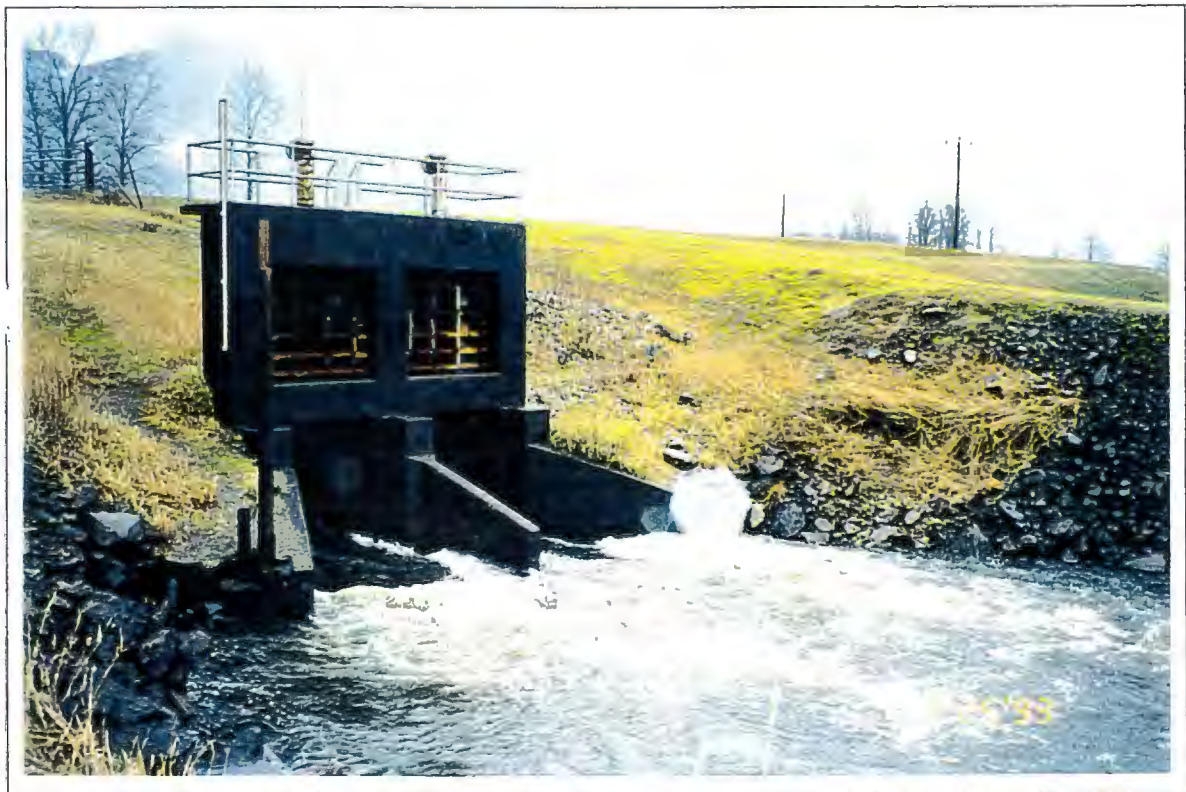
Photo 16: Hammersley pump station: flood box outfall. Note hydraulic jump – possible barrier.
