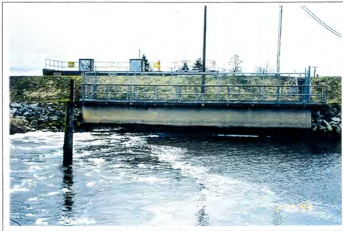
Photo 4: Katzie Slough station: pump and flood box outfall.
