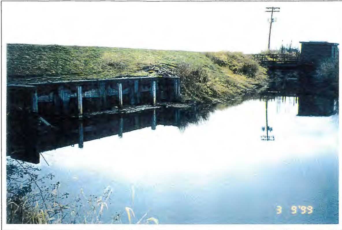
Photo 13: McLean Creek station: flood box entrance (L), pump house (R).
