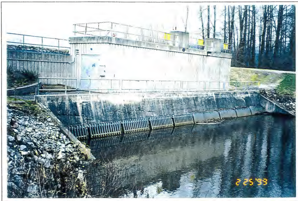
Photo 3: Katzie Slough station: pump intakes (R), flood box entrance (L).
