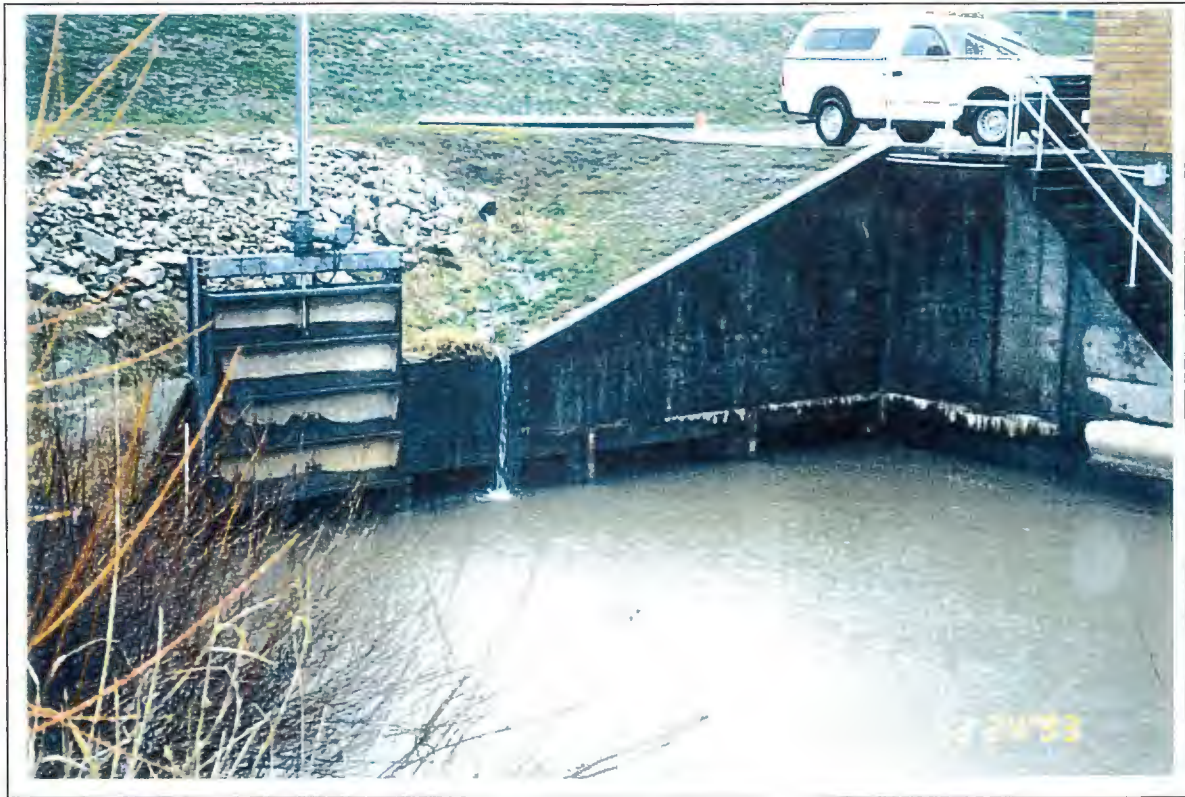
Photo 7: Matsqui Slough station: entrance to flood boxes. Note hydraulic gate and slots for stop logs.
