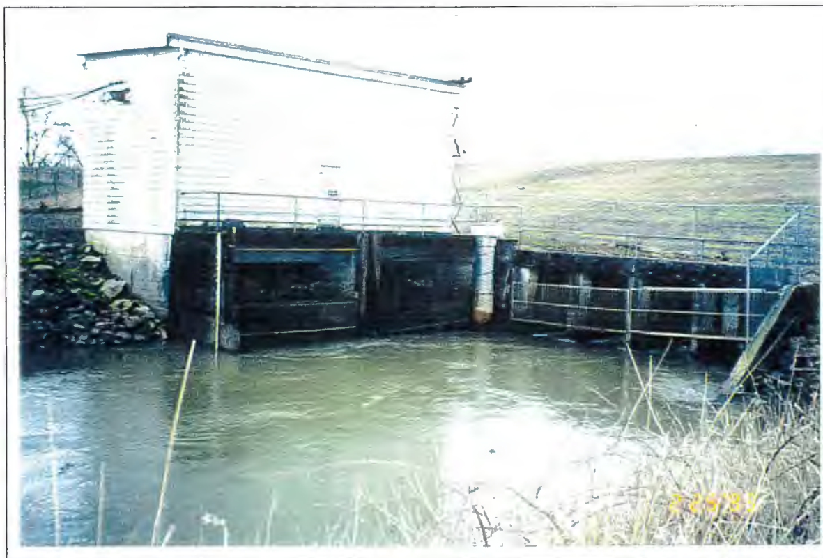
Photo 1: Hatzic Slough station: pump intakes (L), flood box (R).
