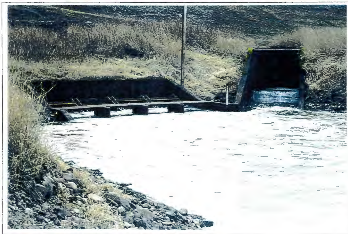
Photo 1: Hatzic Slough station: pump intakes (L), flood box (R).
