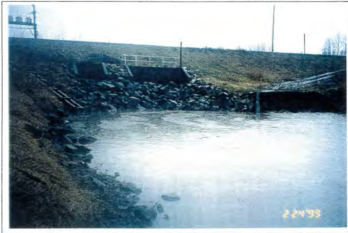
Photo 9: McLennan Creek station: pump (left) and flood box (right) outfalls.
