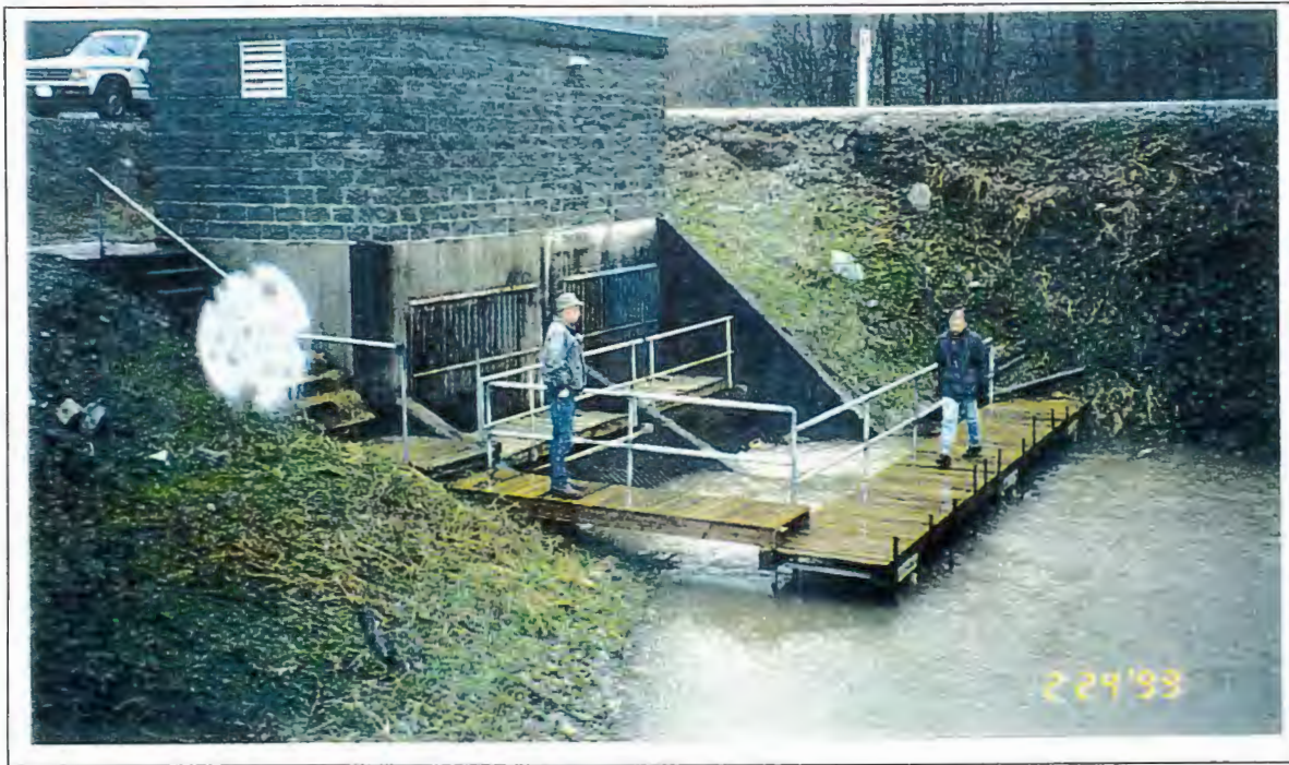
Photo 19: Silverdale station (Chester Creek): walkway to facilitate fish salvage during freshet.
