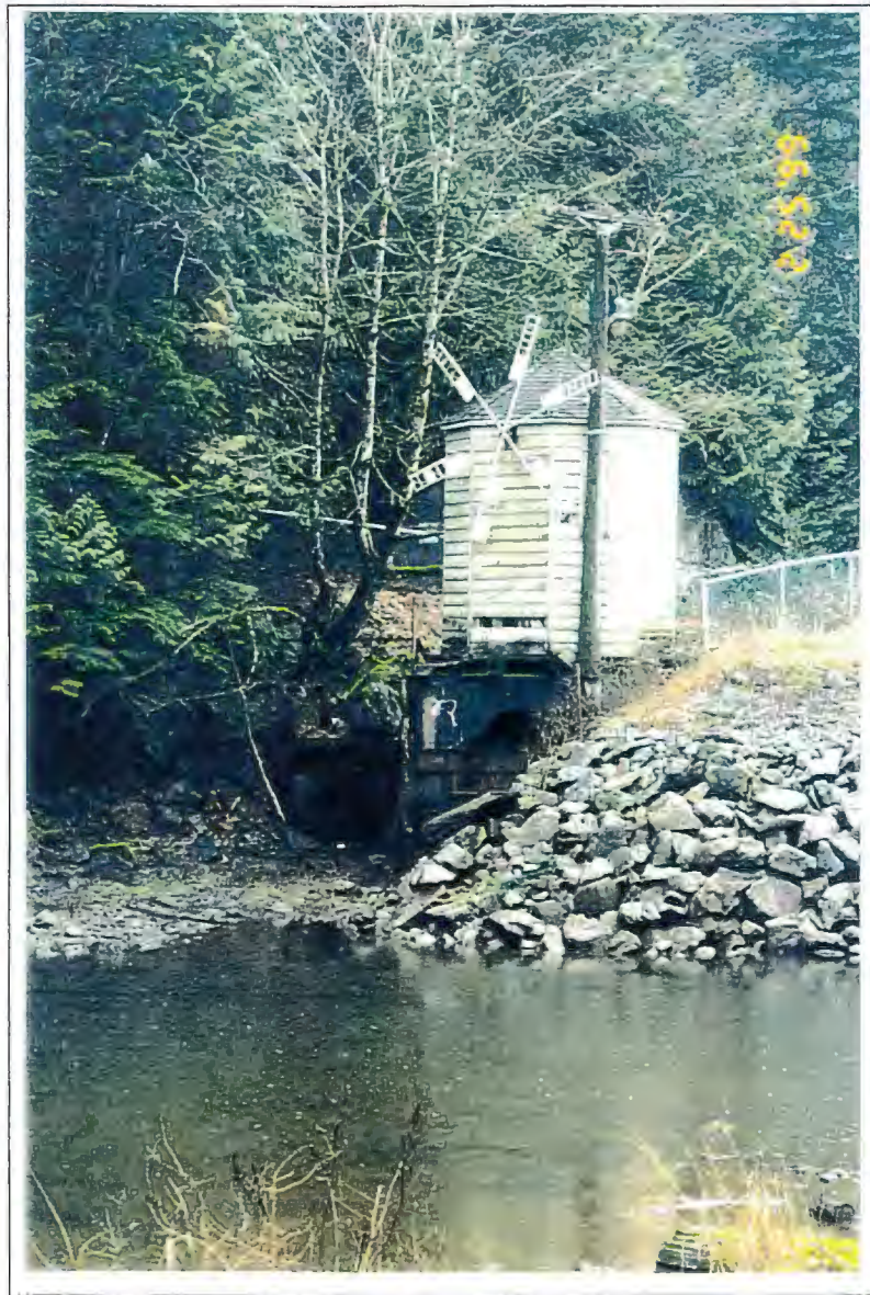
Photo 10: Miami Creek pumping station: old flood boxes under station. Also note the aged screen in front of the sump.
