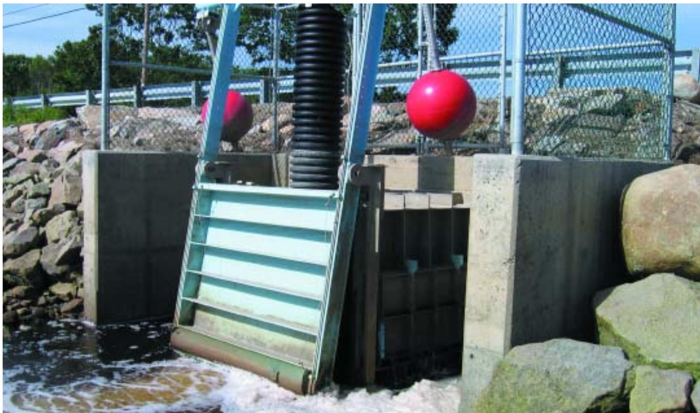
A self-regulating tidal gate that allows fish passage – photo courtesy of Tony Bowron
